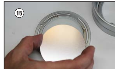
Installing aluminium baffle only under glass (optionally)
